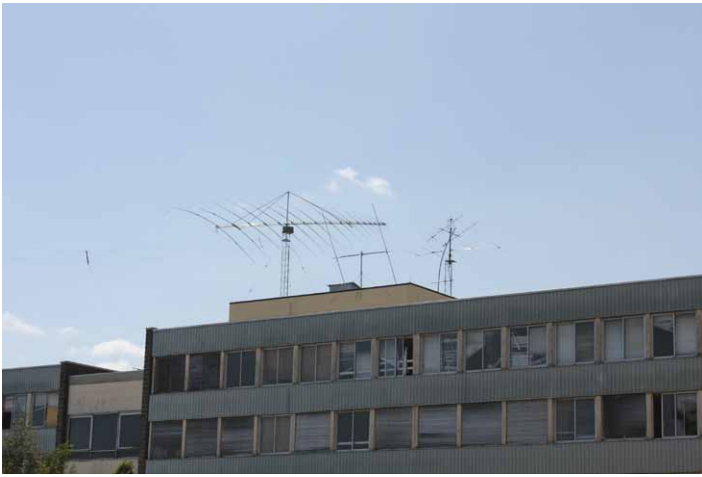
Antennas at ET3AA
